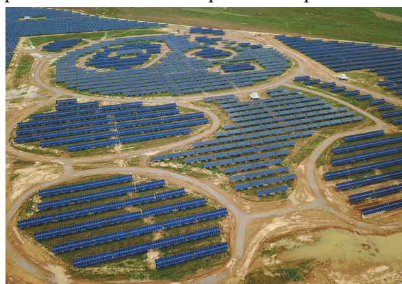
Figure 3: Panda shaped solar installation in Datong, China
