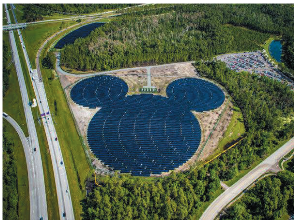
Figure 4: Mickey Mouse shaped solar panel installation in Florida
