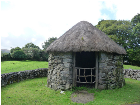
Cornish powder house: the explosives store
