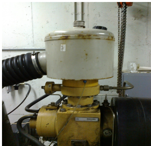
Figure 8. The condenser
