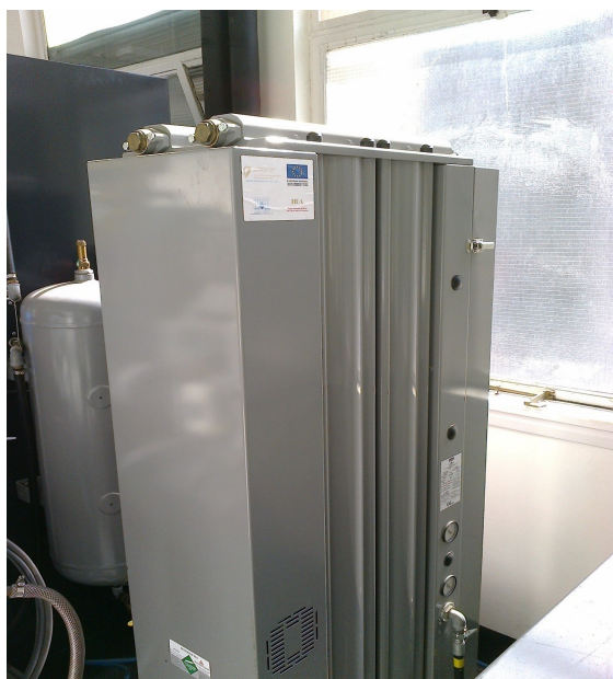
Figure 4. The pressure swing absorber
