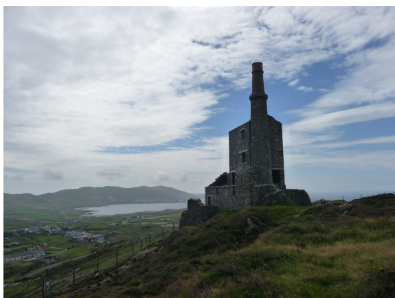
The Mountain Mine engine house at Allihies, looking out over Ballydonegan bay. (see also cover photo)
