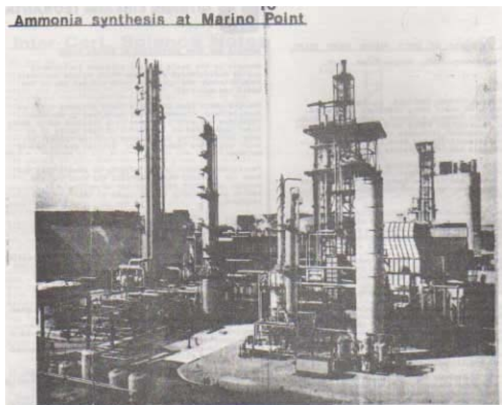
Figure 1 A general view of the ammonia/urea plant complex at N.E.T., Marino Point, Cobh, Co. Cork (Photo: N.E.T.)
