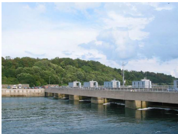
The tidal barrage power station at Rance, Brittany.
