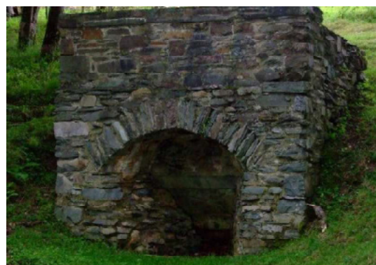
Figure 5: Some typical Irish lime kilns
