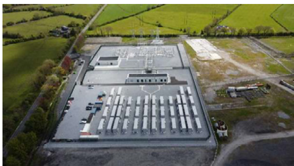
Lumcloon And Shannonbridge 200mw Bess
