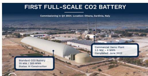
EnergyDome CO 2 batteries in Sardinia. CO2 Battery can cover a large set of use cases due to its long duration, and fast response time, enabling revenue stacking for customers
