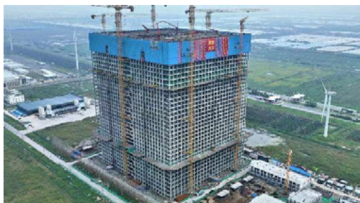
A gravity battery under construction in Rudong, China. Rudong-EVX-Sept-2023-1.jpg (1600×900)
