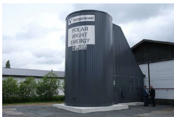
A sand battery recently opened in Finland.
