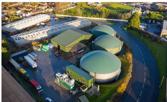
Figure 2: A biogas plant at Lisburn, N. Ireland Biomethane boost: NI biogas plant to power 'green' trucks with food waste - Agriland.ie
